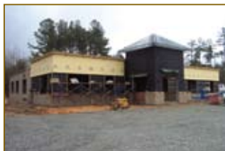
Dogwood Veterinary Hospital Vickers Road, Chatham County
